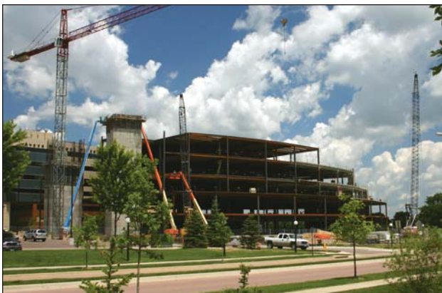
Construction continues on the Avera Cancer Institute in Sioux Falls.
